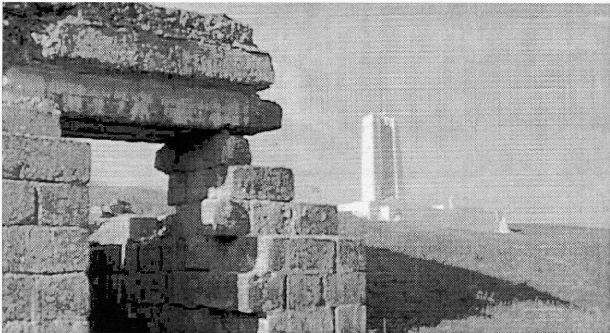
The remains of a German command post on the slopes below the Canadian memorial. No access has yet been affected into the substantial German tunnel systems under Vimy Ridge. They are thought to be at least as extensive as the British workings.
